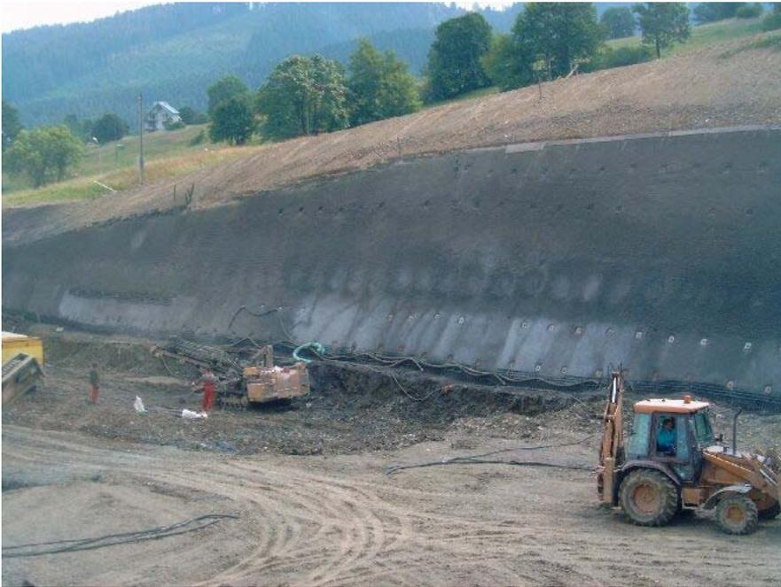
Fig.2 Secured shotcrete wall by TITAN Soil Nails
