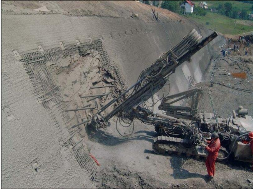
Fig.3 Micropiles TITAN 73/53 for bridge foundation
