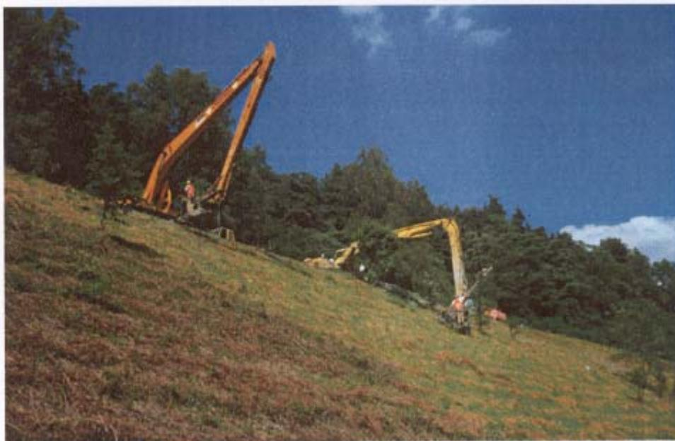
Fig.1 Installing nails from the embankment crown
