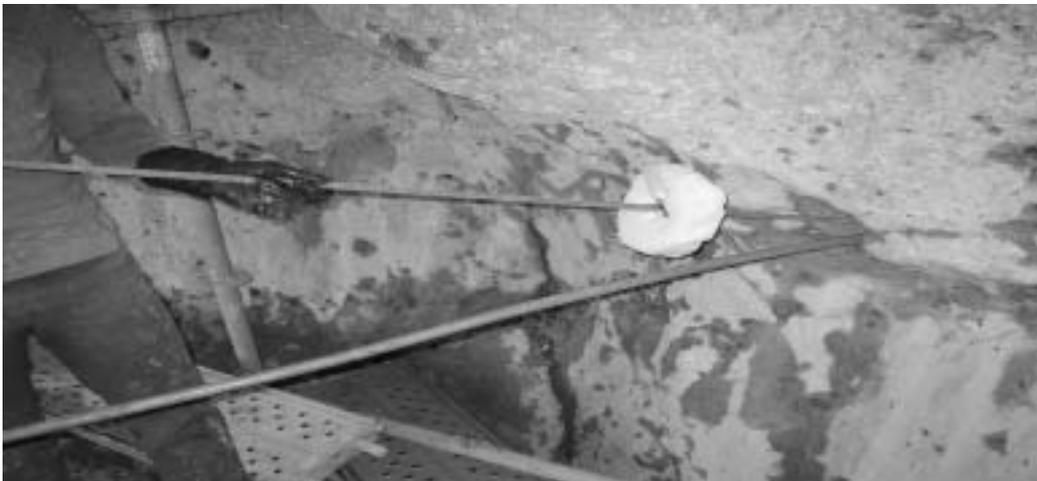
*Inserting of Carbopree® rod 16mm in the rock – Mahon island (ES) soil nailing*
