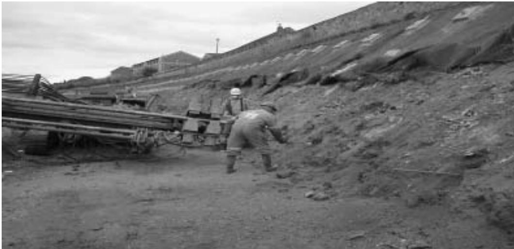
*Inserting 7mt Carbopree® 16mm rod – Sunderland (UK) soil nailing*
