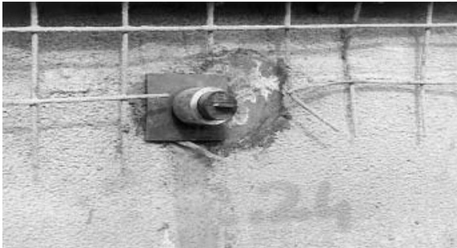
*Conical wedges system with carbon fibre flat bar 40x5mm - London soil nailing*
